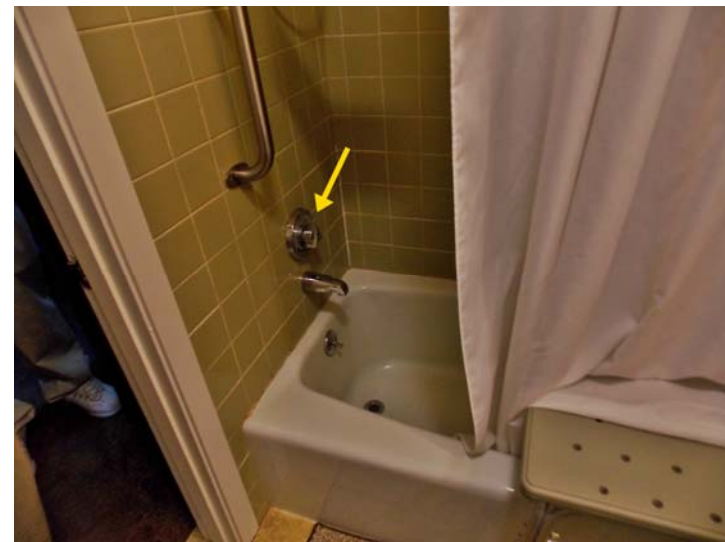
Bathtubs have ceramic tile surrounds and anti-scald mixing valves.
