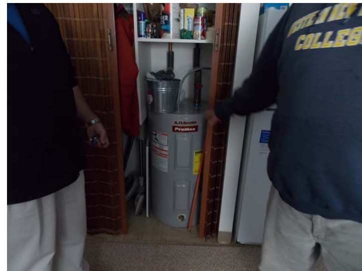
This is a typical electric-heated DHW tank within an apartment.
