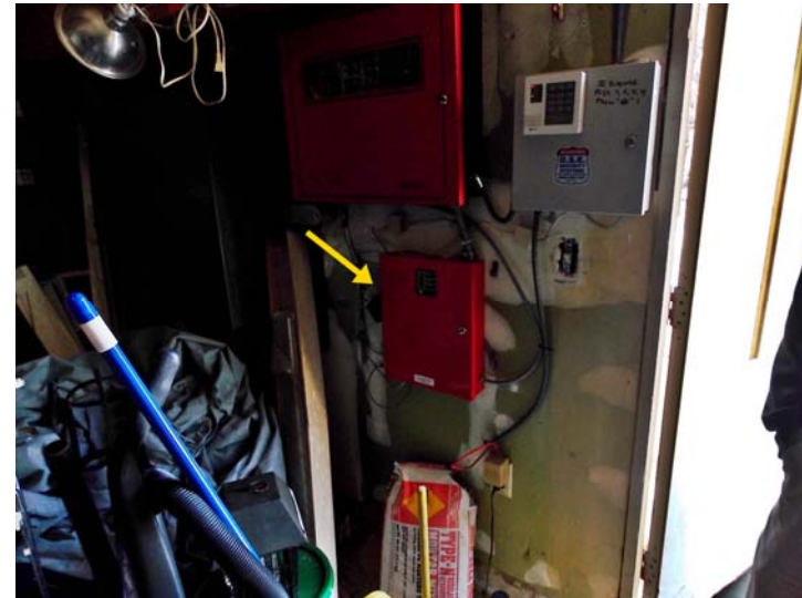
The fire alarm system has been recently upgraded with a newer panel and dialer (arrow).
