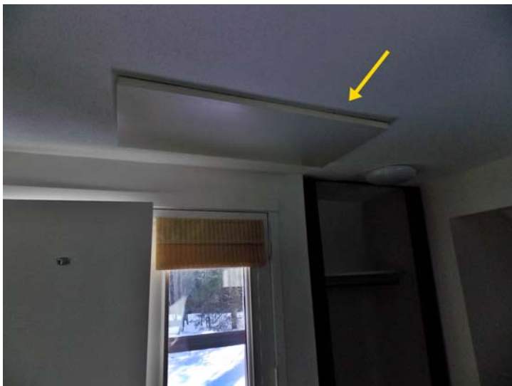
Apartments also have an electric radiant heat panel (arrow) near the rear entrance door.
